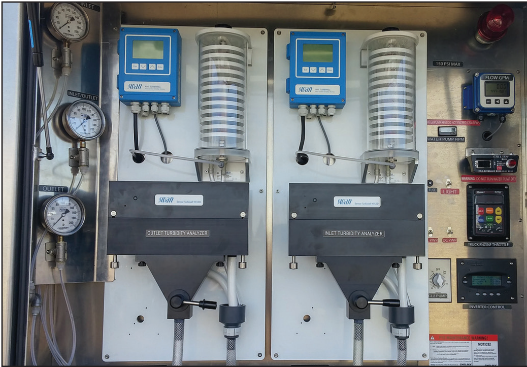
The control panel on the Neutral Output Discharge Elimination System, NO-DES, truck includes meters and gauges to monitor flow, filter loadings, water quality and system performance. Photo courtesy of NO-DES Inc.
