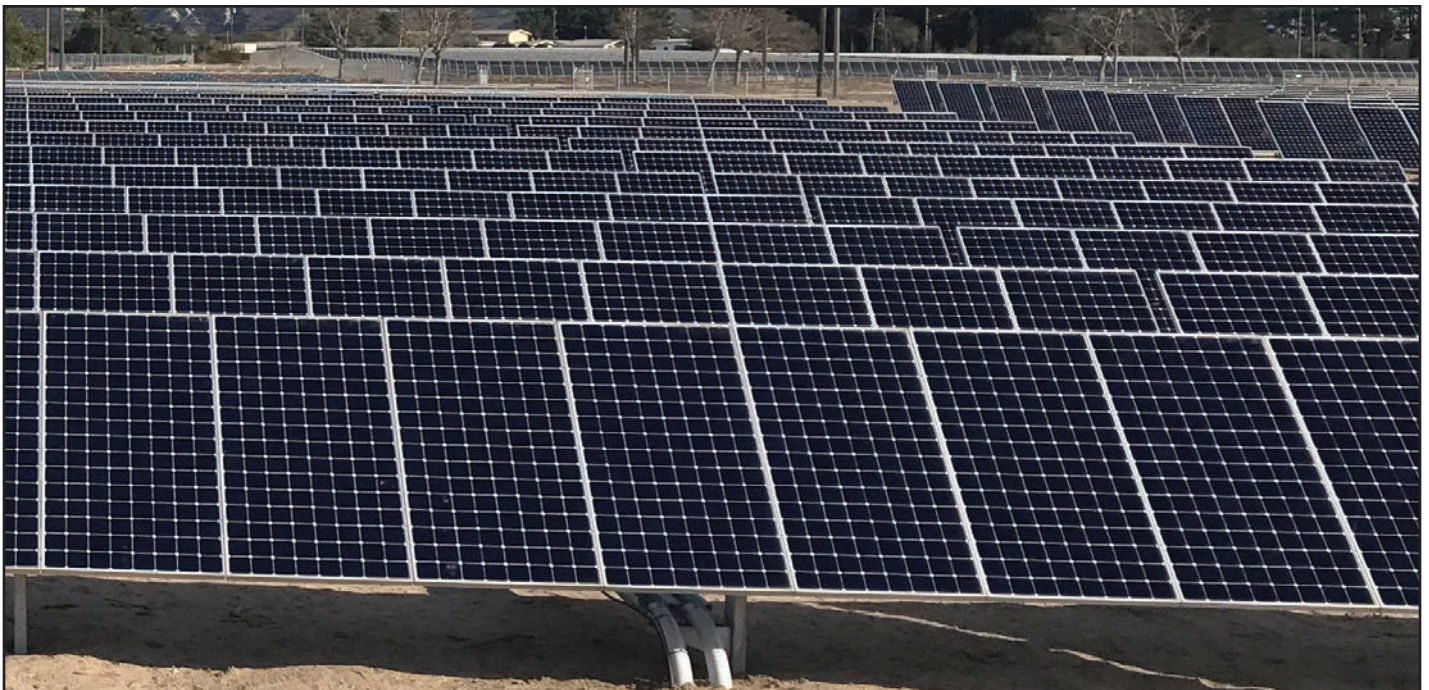
Solar panels stretch across 180-acres, or roughly 163 football playing fields, at the new solar energy facility on Vandenberg Air Force Base, California. U.S. Air Force photo by Airman 1st Class Clayton Wear.
